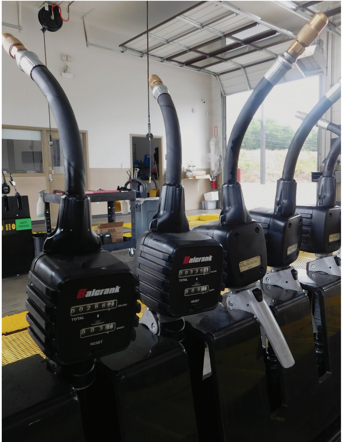
Mechanical Oval Gear Meter Control Handle
